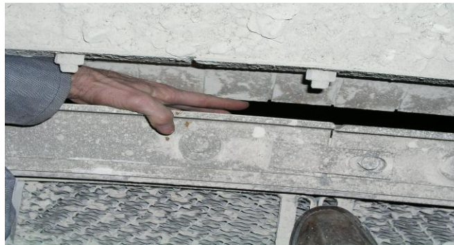
Figure 14, Original Style Circumferential Seal
