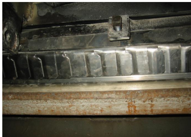
Figure 13, DURAFLEX Circumferential Seal
