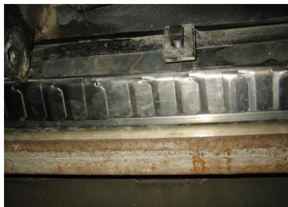
Figure 8, Circumferential Seal
