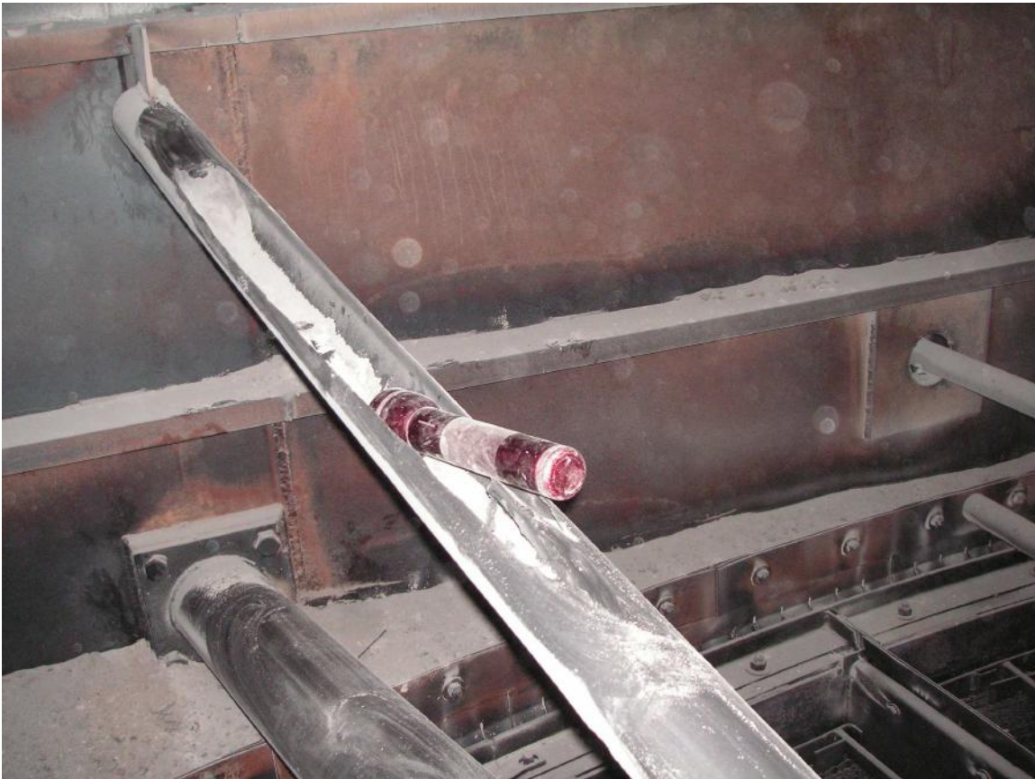
Hot end pipe brace erosion damage
