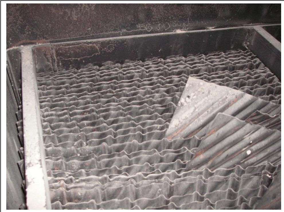
Hot end element damage
