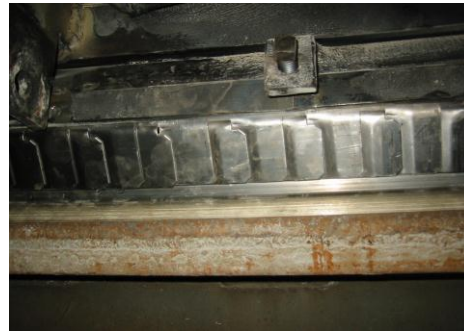
Figure 5, Circumferential Seal
